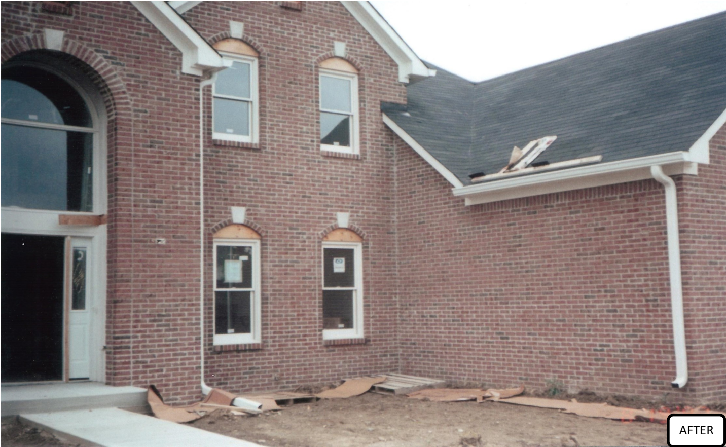
Poorly blended wall with areas of unwanted light brick.
